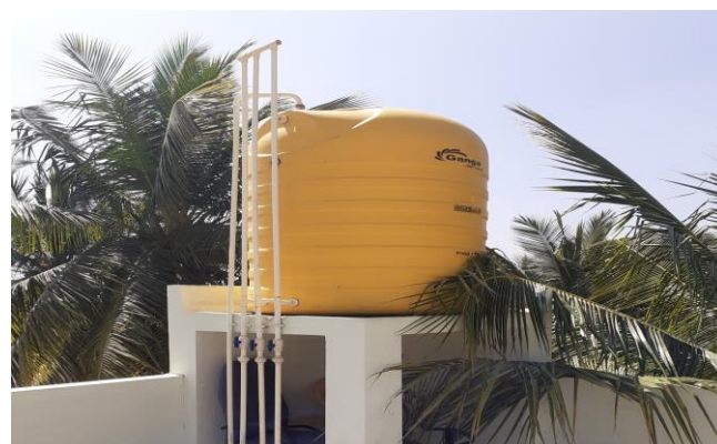
Overhead water tank at GUHPS, Savakanahalli
